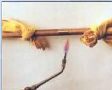
Be sure not to aim the blowtorch directly at the plastic
